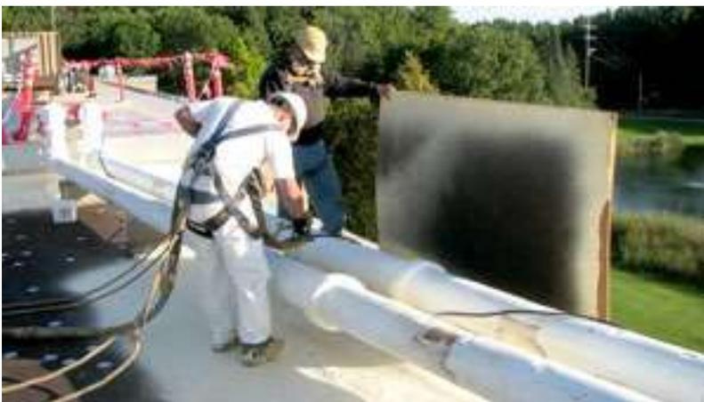
However, the crew could not escape their first item to attack: the old ballasted EPDM system. After removing the old EPDM system, the crew found a rigid board with aluminum facing on it. Because about 80 percent of this layer was dry, they merely had to remove the wet parts and replace them with one-and-a-half-inch iso board. The Kohls crew attached the new recovery board over the insulation with three-inch plates and metal fasteners, which ranged in size depending on the depth of the
